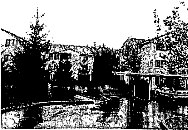
The Park at Forbes Creek Apartments
