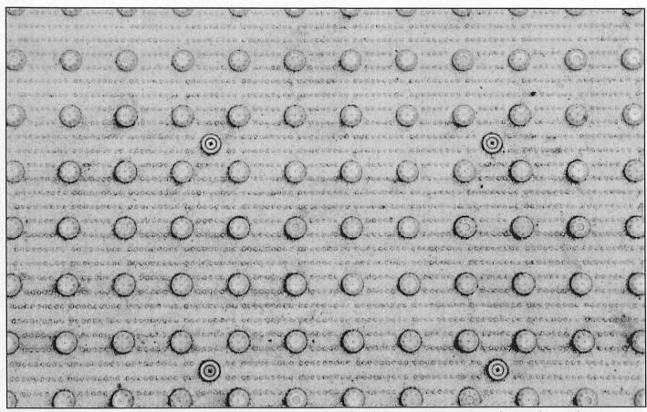
A tactile warning mat uses texture to alert the visually impaired that they are about to enter the roadway. These mats have been a common feature of sidewalk access ramps since the 1990 passage of the Americans with Disabilities Act.
