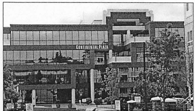
This building uses both horizontal and vertical modulation to add interest and reduce its visual bulk.
