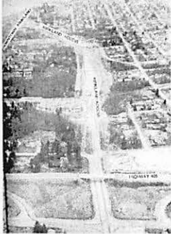
Construction of NE 85th Street
