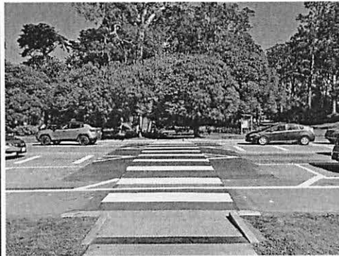
Example of a raised pedestrian crossing at a midblock intersection.
