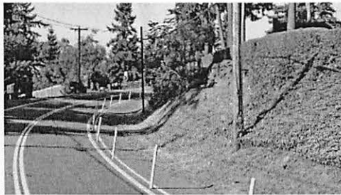
Buffered climbing lanes have already been installed along uphill portions of Juanita Drive (above).
