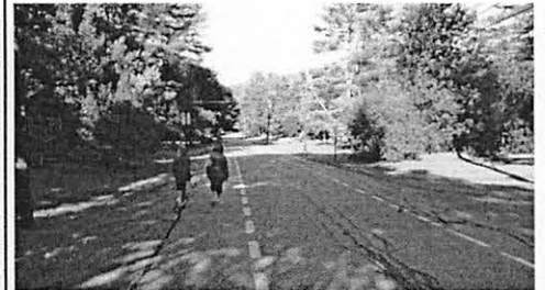
Example of an advisory shoulder using paint as a visual buffer
