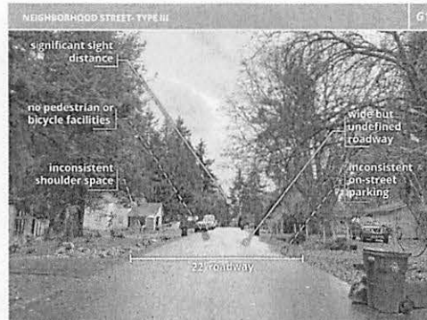
Above: Example of a Type III neighborhood street in the Holmes Point Overlay Area.
