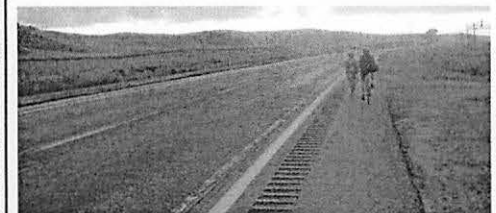
Example of a shoulder separated from the roadway with a rumble strip
