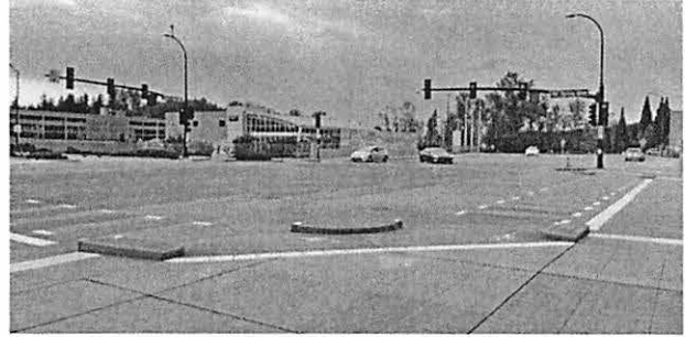
Figure 1.52: Protected intersection in Bellevue (City of Kirkland).
