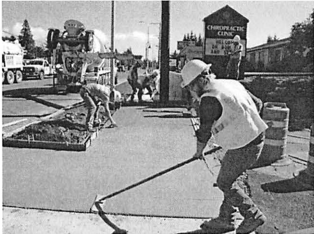
Figure 1.44: Sidewalk construction project on NE 85th St (City of Kirkland).
