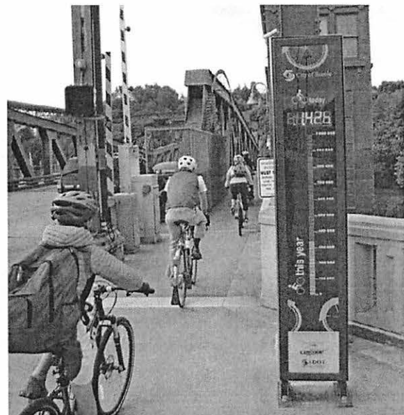
Figure 1.17: Bicycle counter on Seattle's Fremont Bridge ( Puget Sound Business Journal ).
