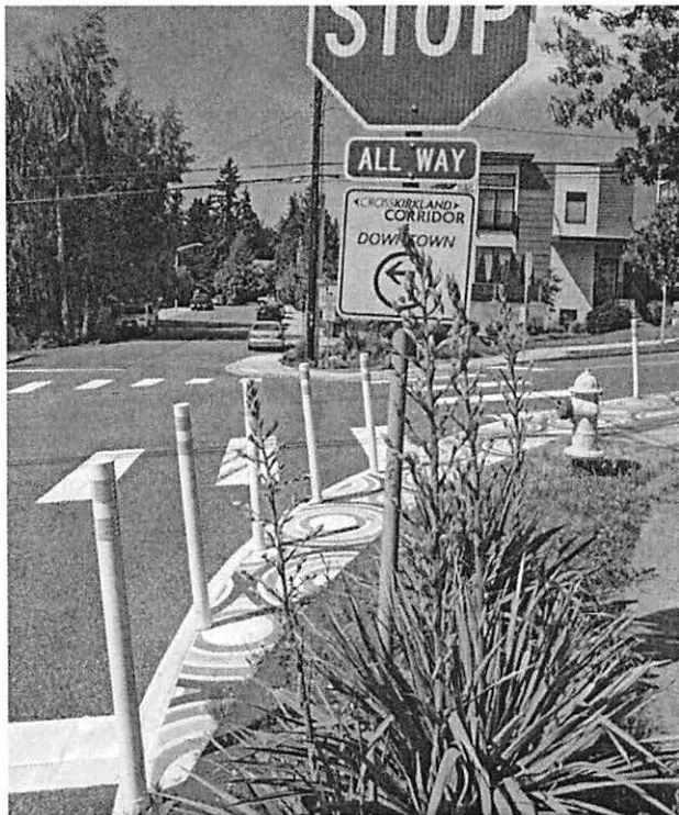
Figure 1.9: Curb bulbout with delineators and a CKC wayfinding sign at intersection of 114th Ave NE and NE 87th St (City of Kirkland).
