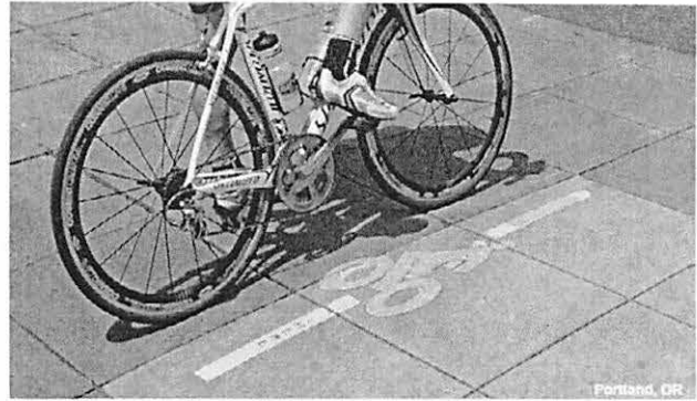
Figure 1.12: Loop bicycle detection system in Portland, OR (NACTO).
