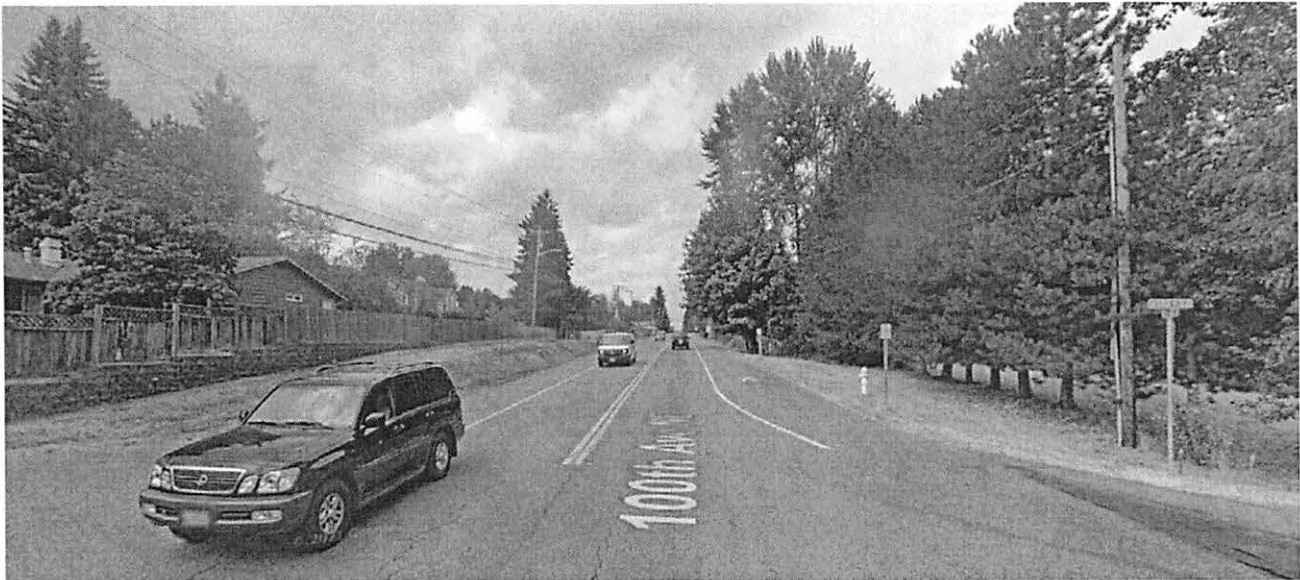
Figure 26. Unprotected crossing on 100th Ave in North Kirkland. This is a long, straight and level section without traffic control devices and little separation of modes (Google Maps 2021).
