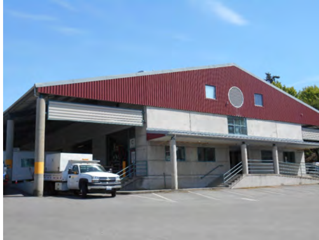
City of Kirkland Public Works Maintenance Center Extension
