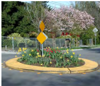
Example of traffic circle installed for slowing down vehicle speed
