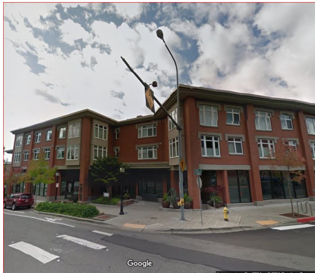
Intersection at 7th Avenue and Market Street
