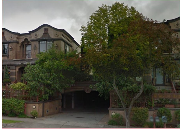
Office Development on Market Street
