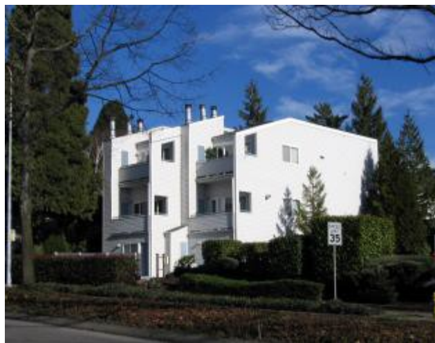
Multi-family Development on Market Street
