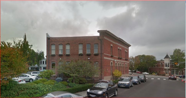
Sears Building at 701 Market Street
