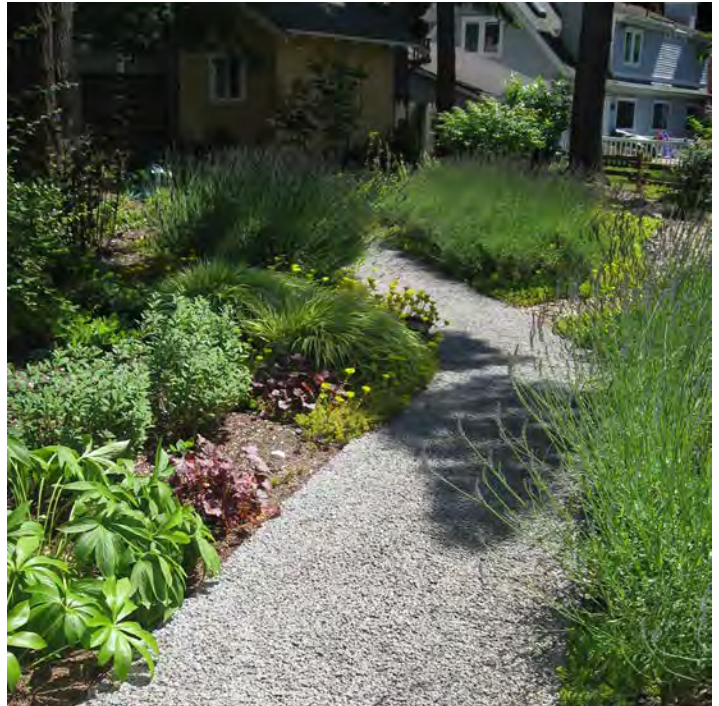
Pervious paving at a development in Kirkland.
