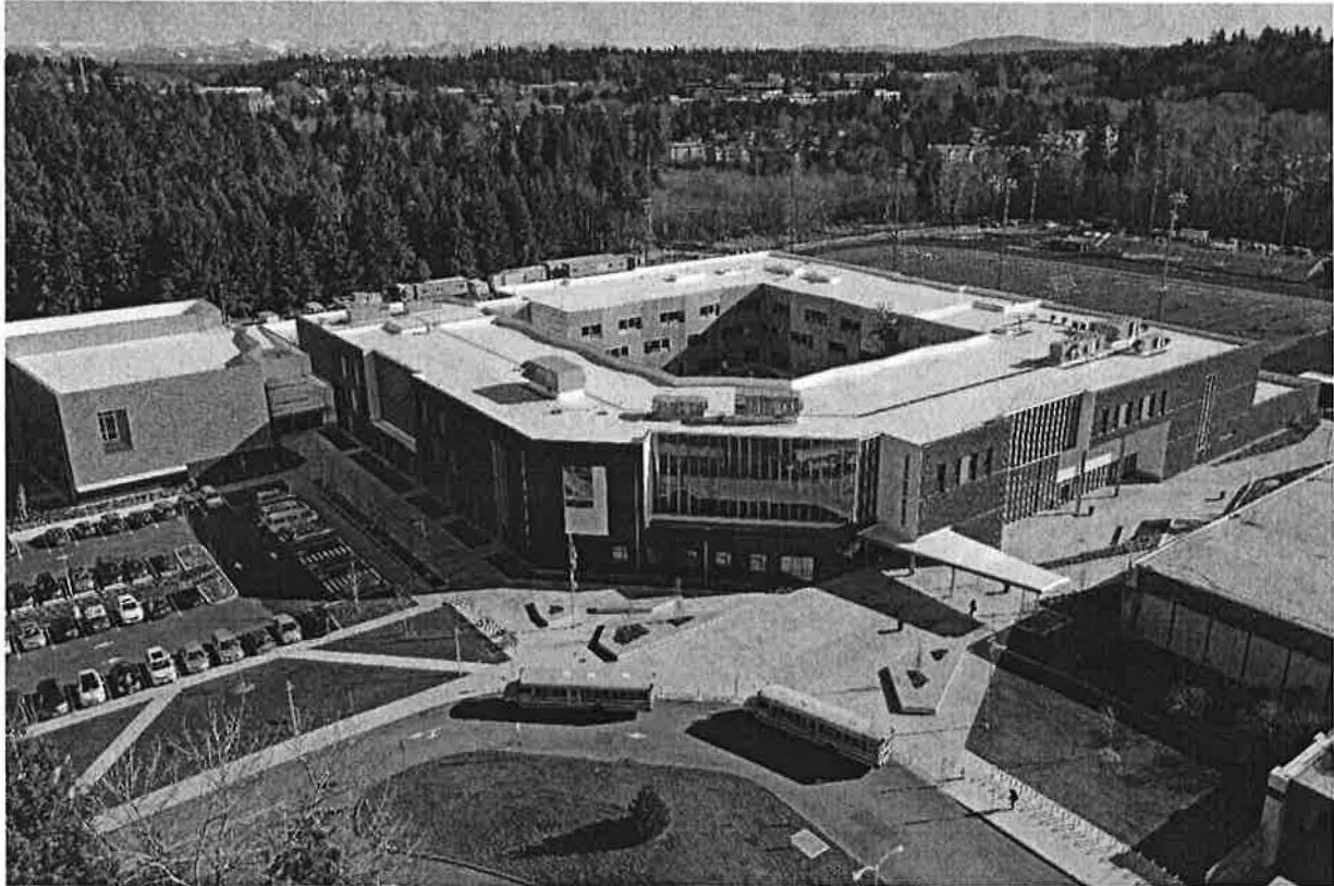
Juanita High School – Phase II To Open Fall 2020
