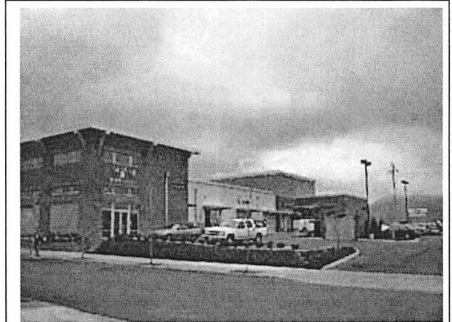
Figure 17. Encourage developments to place parking lots to the side or rear, as accomplished here
