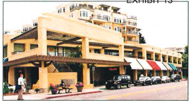
Horizontal modulation elements: canopy, brick banding, and window details.
