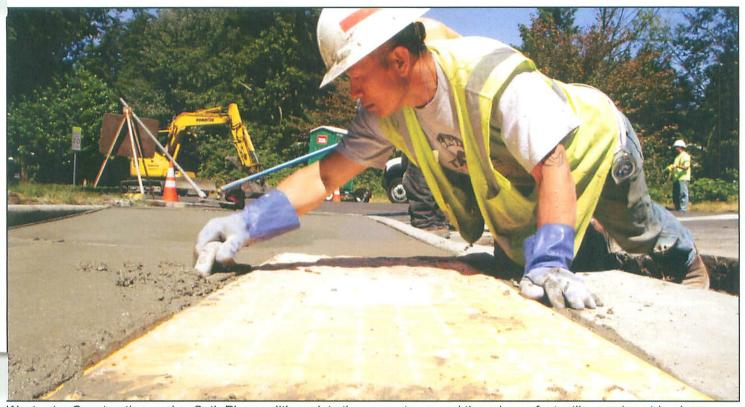
Westwater Construction worker Seth Phonpadith sculpts the concrete around the edges of a tactile warning strip along 100th Avenue Northeast, north of Northeast 125th Street. These tactile warning strips tell the vision-imparied they are about to enter a traffic zone.
