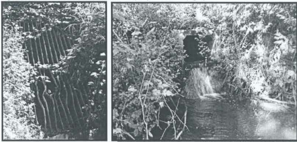
Figure 1 – 100th Avenue NE Culvert Inlet (left) and Outlet (right)
